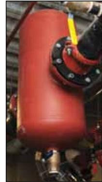
was particularly impressed with the Taco 4900 Series separator and the fact that it didn't require any set-up due to the fact that it comes with a factory installed automatic vent on top.
