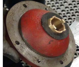
Gasket around Bearing Spacer
