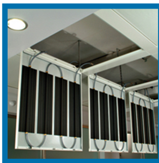
Ceiling radiant cooling panels.
