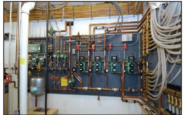
Taco RMBs have just four pipe connections, are quick and easy to install, and save space on mechanical boards. Taber described installing and wiring the RMBs as “so simple. Very easy to lay-out, plumb and wire.”
