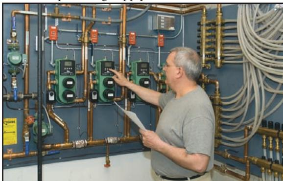
Homeowner/system installer Steve Taber sets parameters for one of four Taco Radiant Mixing Blocks. Each device offers complete injection mixing, combining a variable speed injection mixing control, injection circulator, system circulator and air elimination in a single unit.
