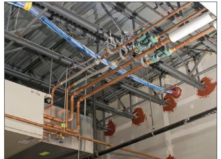
Nowak then finalized the design, employing just over 100 LoadMatch circulators and McQuay fan coils, and added a thermal ice storage system to save additional energy.
