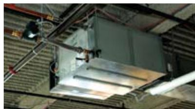
The building contains 72 FHP heat pumps, each with a Taco LoadMatch pump.
