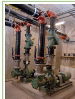
Taco FI series pumps and Plus Two Multi-Purpose valves in the Ascent mechanical room.
