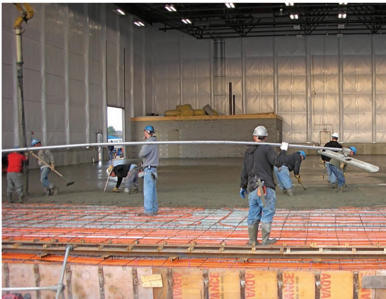
Al Hill Plumbing techs lay tubing for radiant heat in an airplane hangar.
