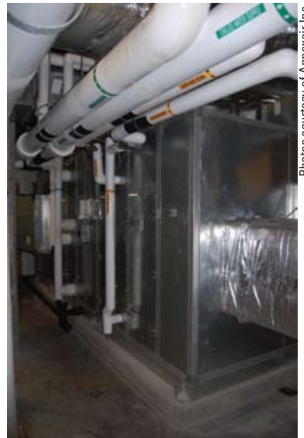
The energy-recovery ventilator installed in the penthouse equipment room.
