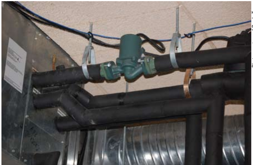
One of many load-matching pumps installed at Proximity Hotel.
