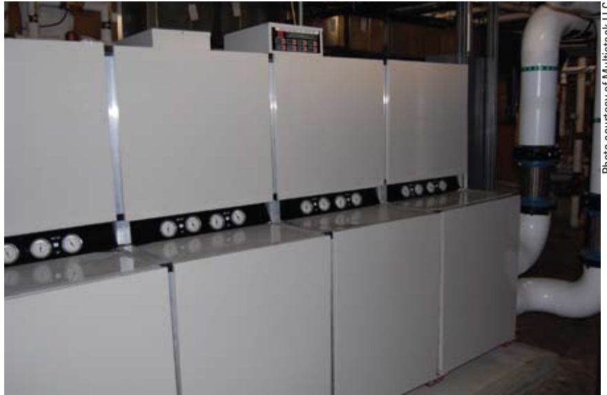
The 200-ton modular scroll-chiller system at Proximity Hotel.
