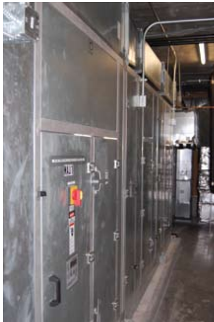
The energy-recovery ventilator installed in the penthouse equipment room.
